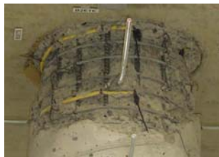
Figure 6. Before (left), and after (right) loose concrete chipping
