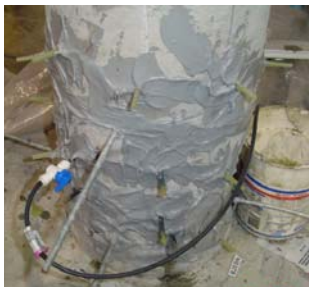
Figure 7. Epoxy injection
